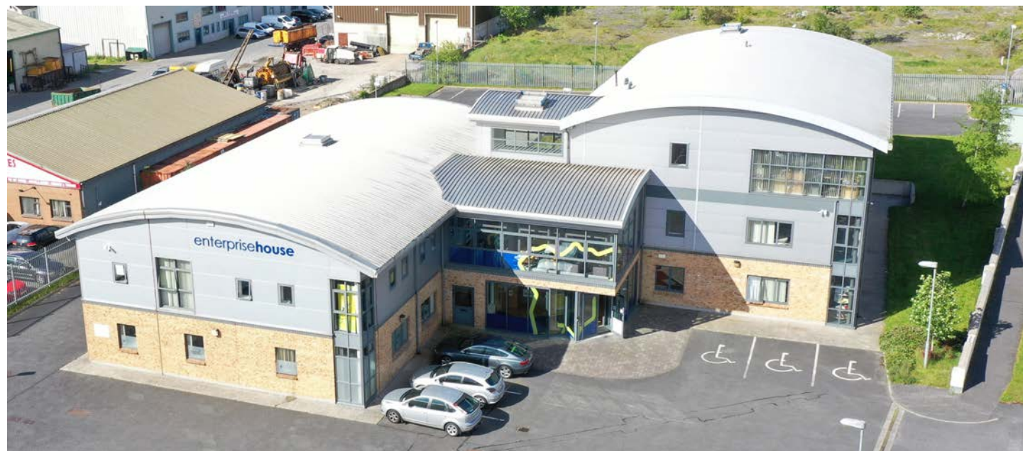
Enterprise House, O’Brien Road, Carlow – part of the Connected Hub Network
