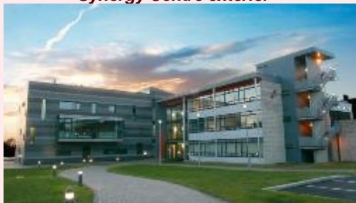
Synergy Centre exterior
